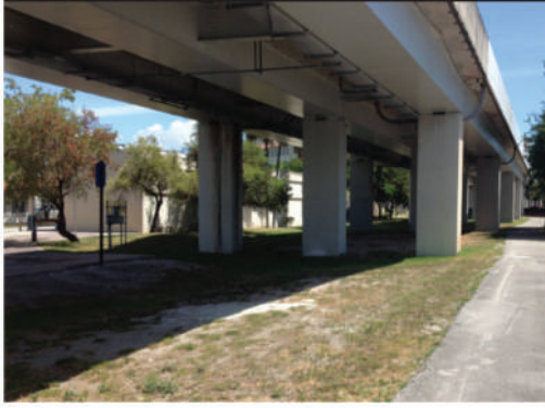
Underline Douglas Metrorail Station Before
