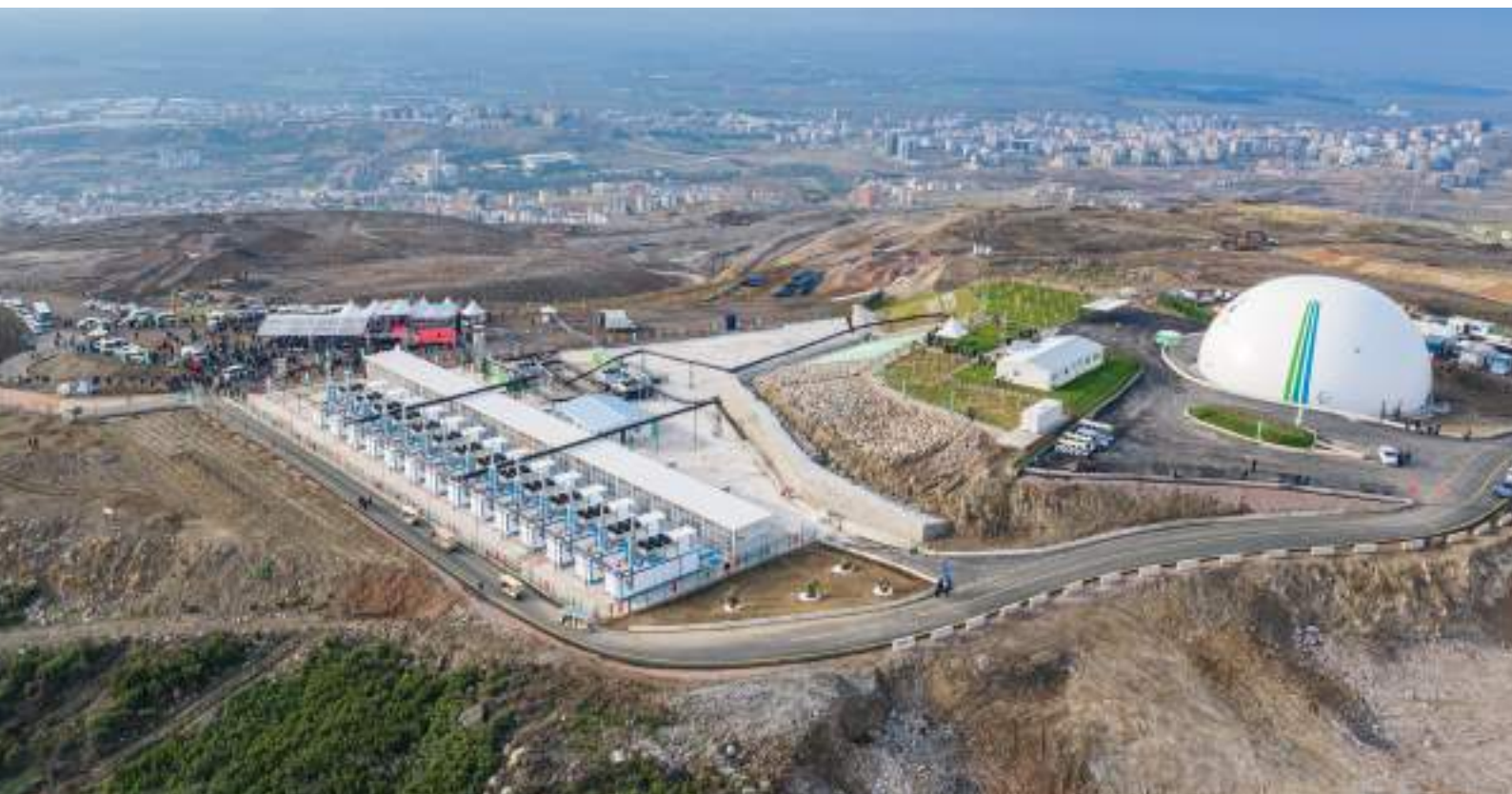
Harmandalı Solid Waste Landfill and Biogas Facility
