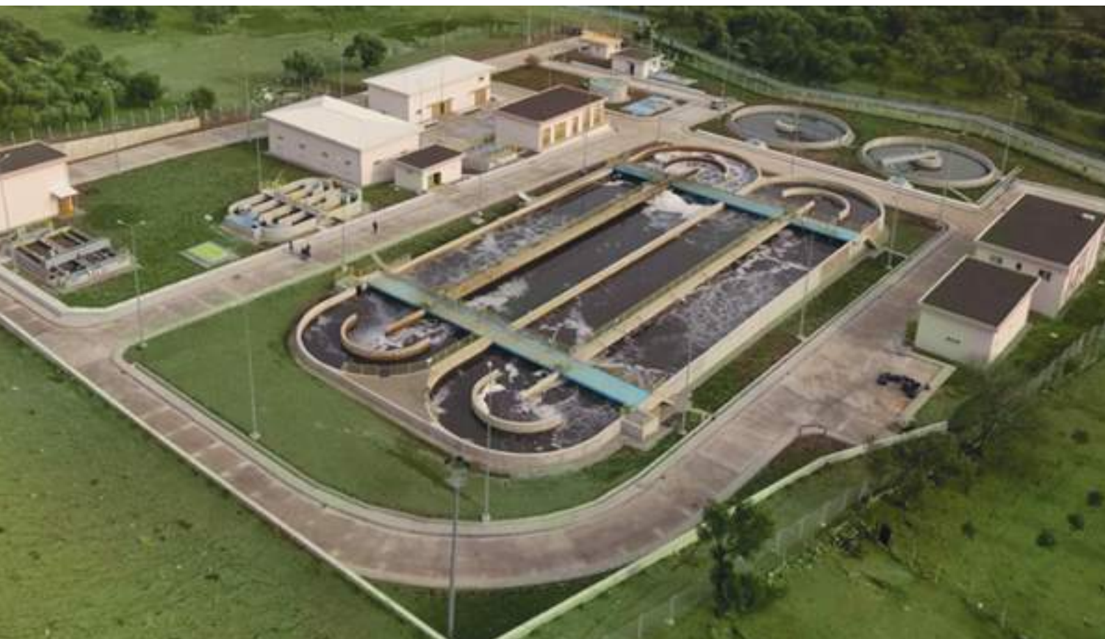
Çiğli Wastewater Treatment Plant
