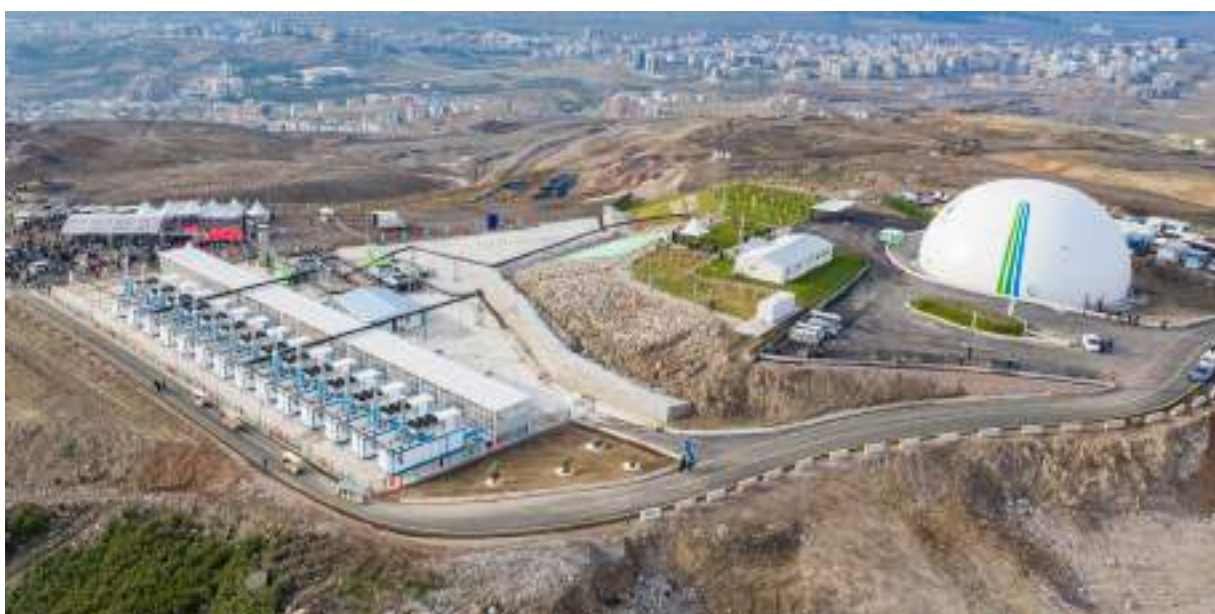
Harmandalı Harmandalı Solid Waste Landfill Facility
