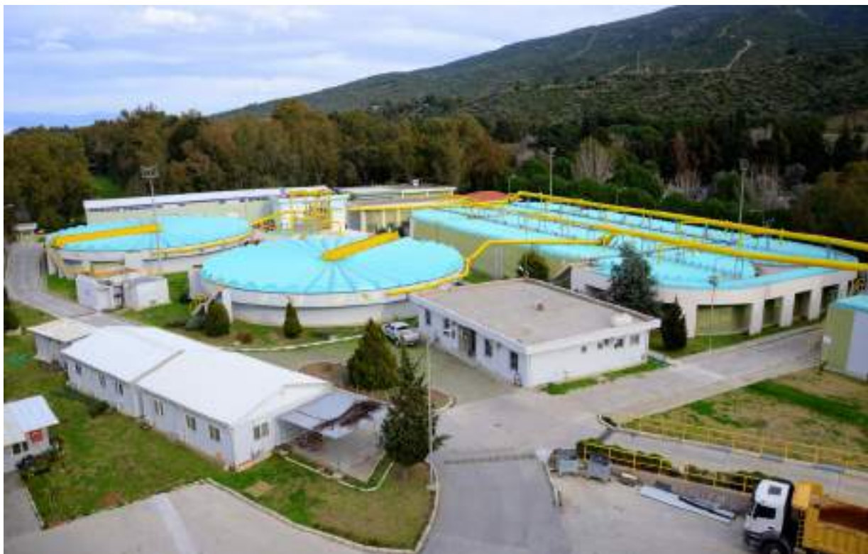
Southwest Advanced Biological Wastewater Treatment Plant
