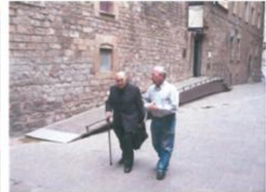
Adjustment of entrance to an old building, steps on one side and ramp on the other. Could be better even with handrail on wallside of ramp.
