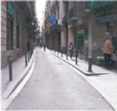
Lowered steps to sidewalks, and no obstacles
